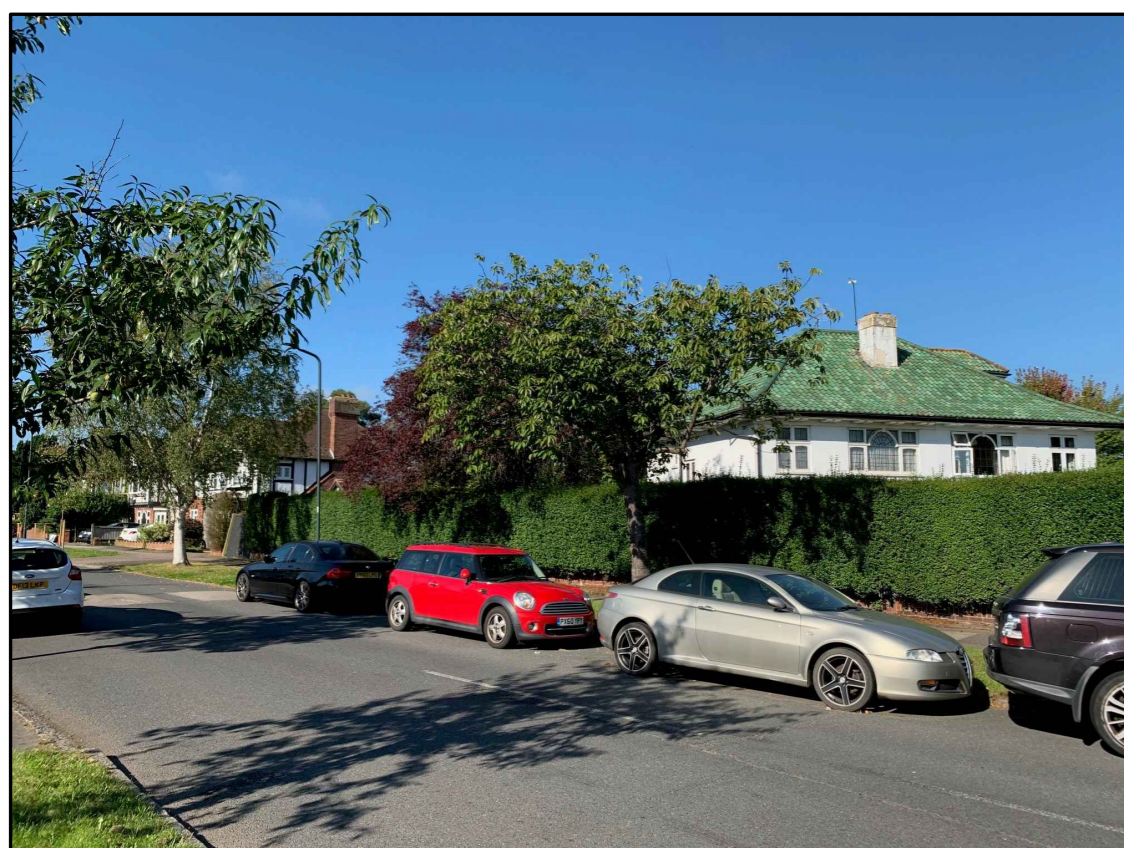
EXISTING FRONT CORNER PHOTO
