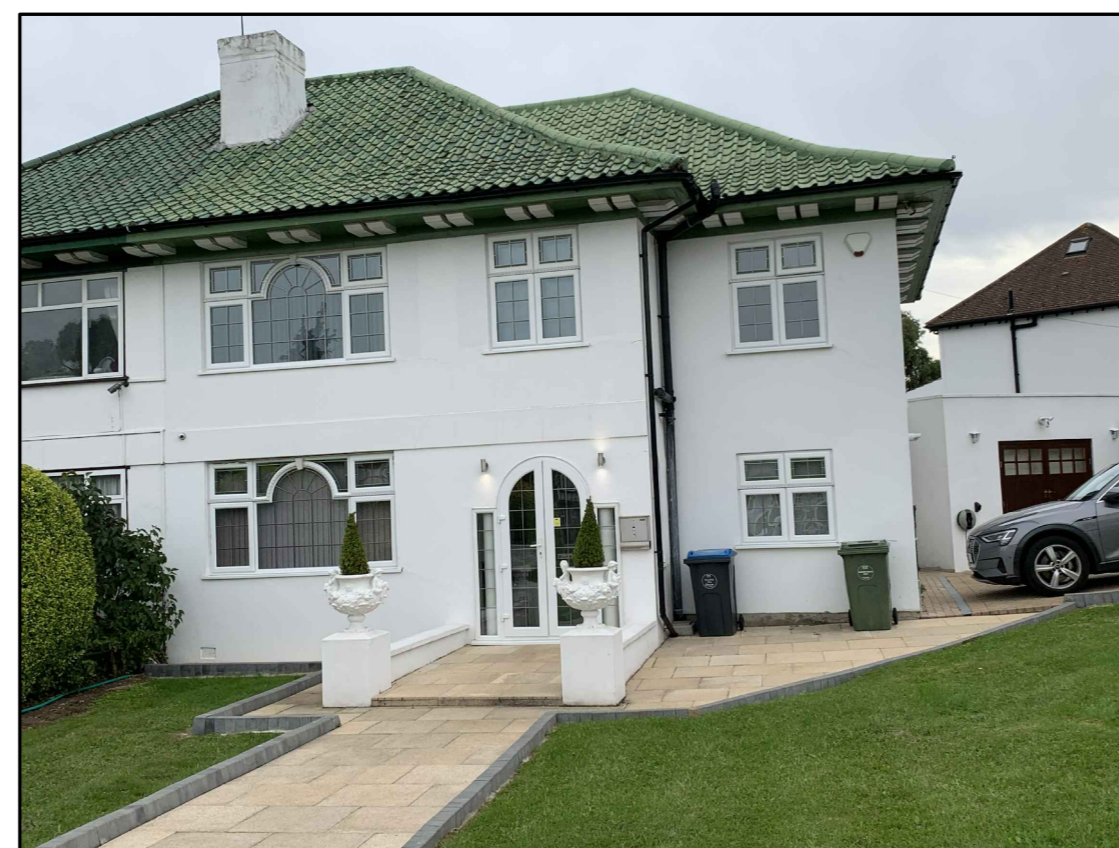
118 PAXFORD ROAD, WEMBLEY, HA0 3RH- EXAMPLE OF FRONT PORCH
